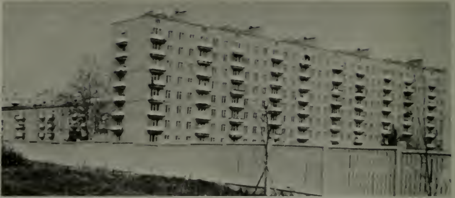
A typical Moscow apartment building.
